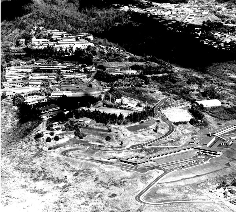
Construction of the lower campus. No date given.
